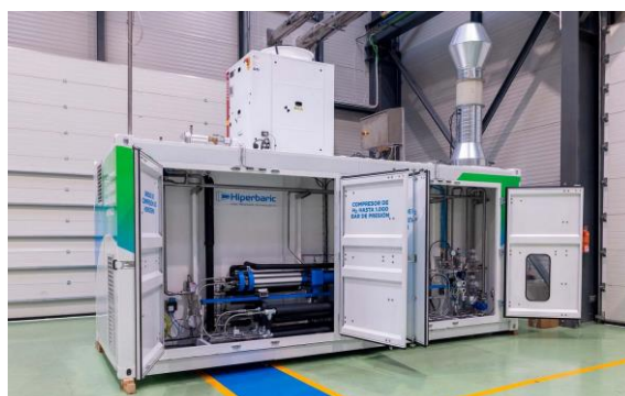
Obr. 51 - Kompresní stanice Puertollano Hydrogen Station [41]
